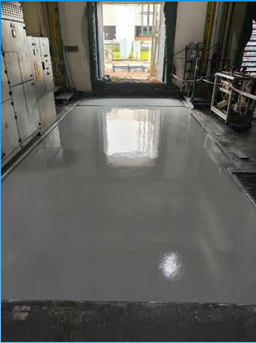
Floor Levelling with Epoxy Lining
