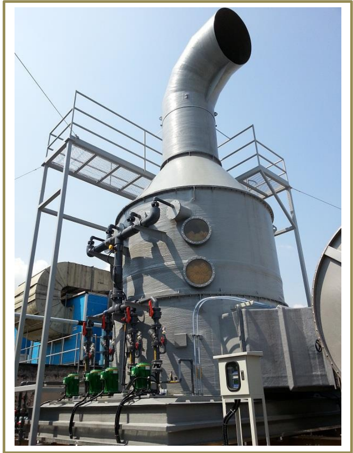
Vertical Scrubber Installation for a semiconductor plant
