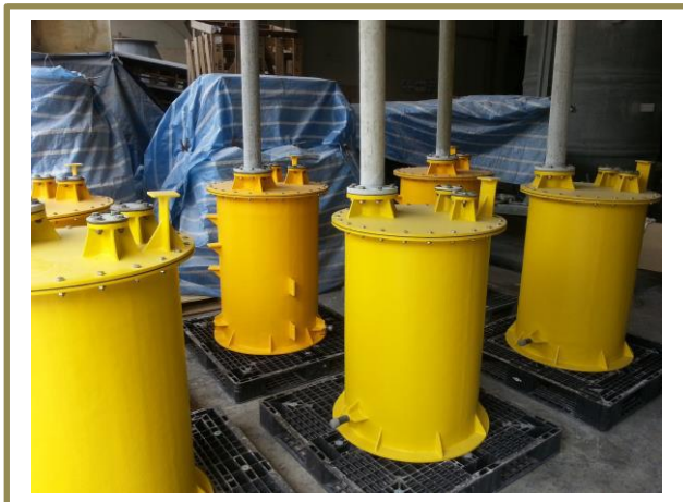
Chemical storage tanks undergoing hydrostatic test
